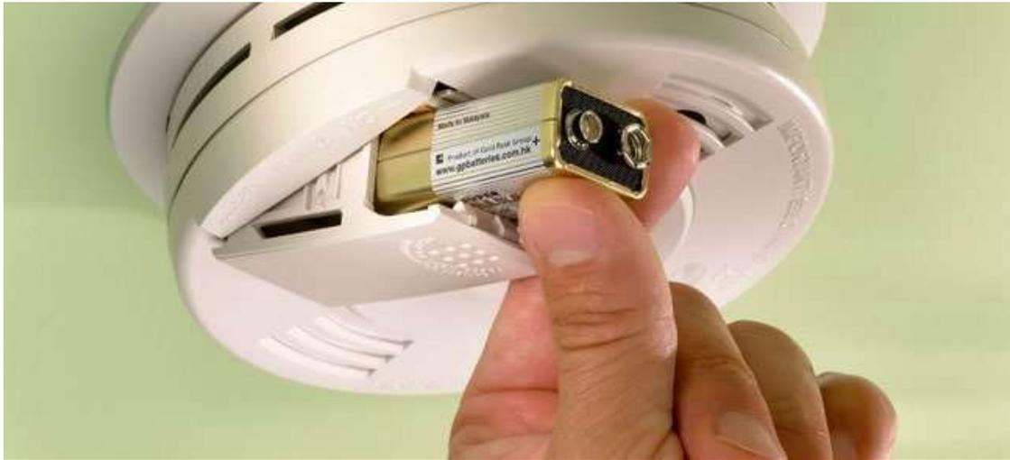
Check the batteries in your smoke and CO detectors checked according to manufacturer's specifications.
