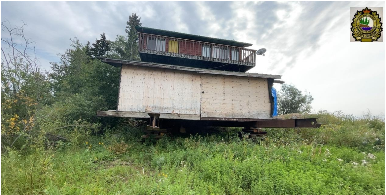
Photo of the structure to be removed.
