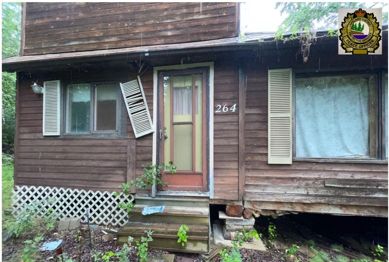
Photo of the structure to be removed.
