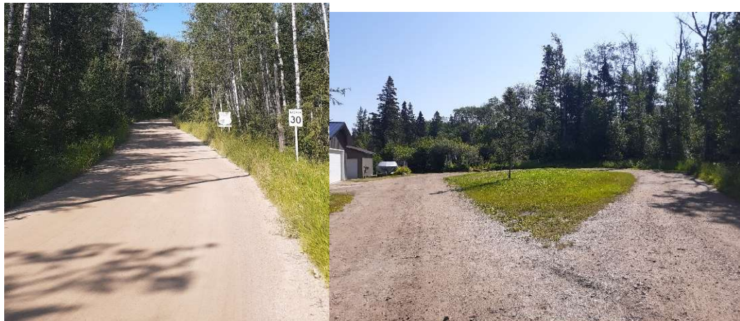
Figure 3: Left picture showing narrow road driving surface and unmaintained shoulder. Right picture showing large turnaround .
