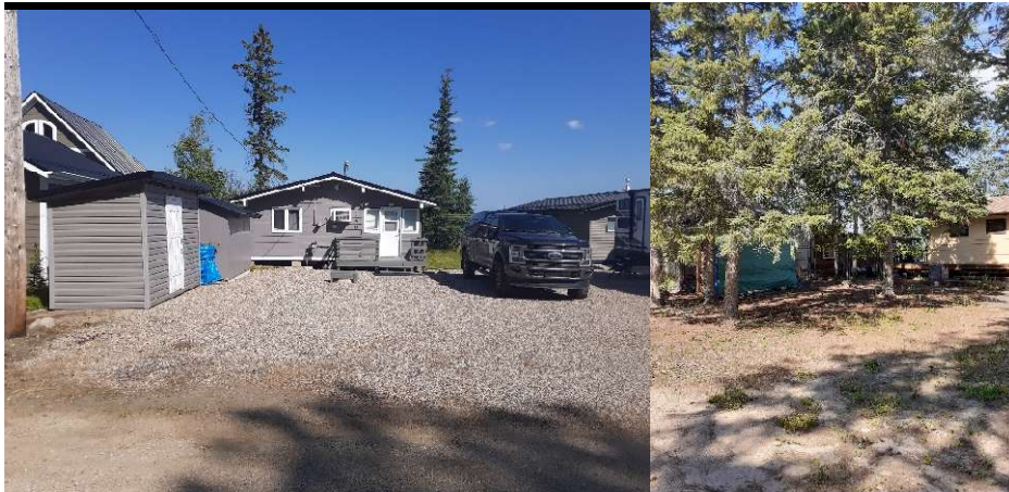
Figure 10: Houses on left shown with clean asphalt, minimal vegetation against structure. Right picturing showing pruned conifers.
