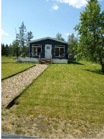
Figure 9: Houses on left shown with clean gravel walkway, minimal vegetation against structure and skirted deck area.
