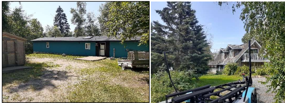
Figure 3: Left picture showing a clean (no leaf litter) asphalt roof. Right picture showing cedar shake roof.
