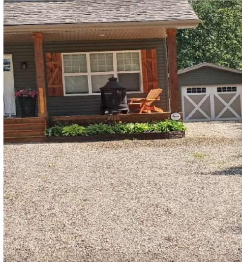
Figure 7: Firepit made of steel mesh that should be moved off of deck to the gravel area before use and away from the structure.
