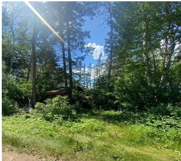
Figure 4: Overgrown vegetation too close to structures.
