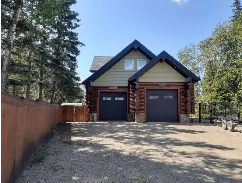
Figure 7: Houses on left shown with clean asphalt, log construction, minimal vegetation against structure and gravel right up to the home.
