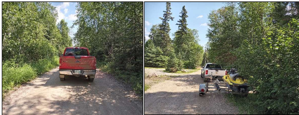
Figure 3: Left picture showing narrow road driving surface and unmaintained shoulder. Right picture showing minimal available driving surface when vehicles parked on edge of road.
