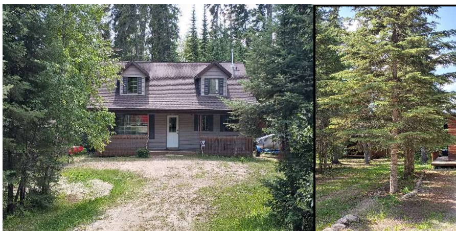
Figure 11: Houses on left shown with clean asphalt, minimal vegetation against structure. Right picturing showing pruned conifers.
