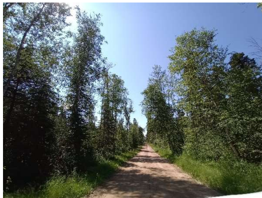
Figure 3: Left picture showing narrow road driving surface and unmaintained shoulder.
