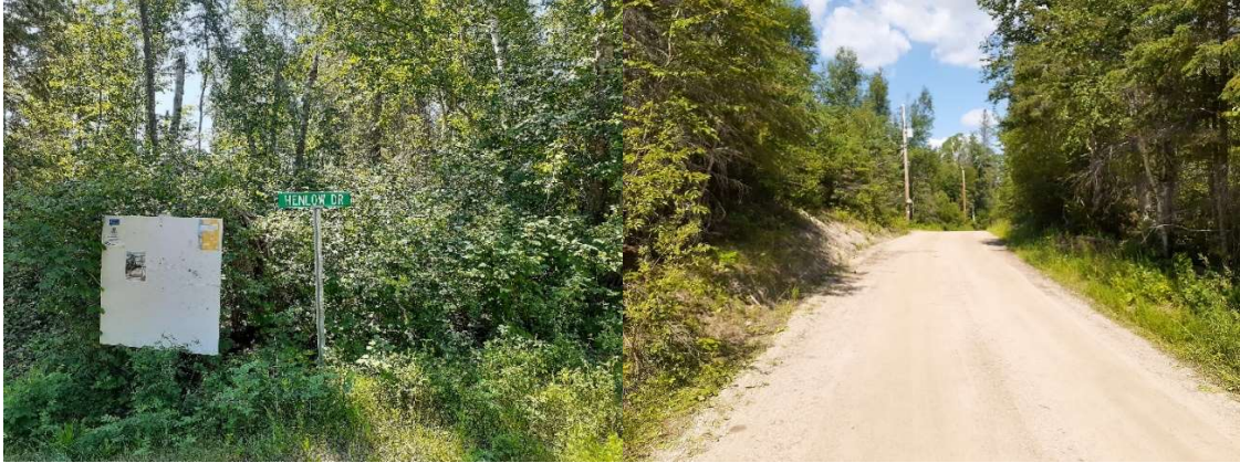
Figure 2: Picture shows metal reflective street signs at subdivision entrance. Right picture showing narrow road with unmaintained shoulder.
